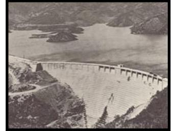
increased the dam's height by twenty feet, no changes were made to its base width. As a result, the intended safety margin for structural stability decreased significantly.
