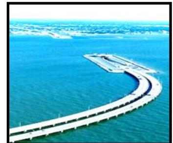
dredged for other parts of the project. In the aerial image, we can see the island as a graceful white crescent in the water. The Oresund Bridge is a cable-stayed bridge. In this kind of bridge, a series of strong steel cables attach the bridge deck to high towers called pylons that support its weight
